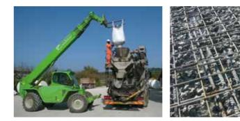
Due to the deep thickness of castings, the latter must always be reinforced.
